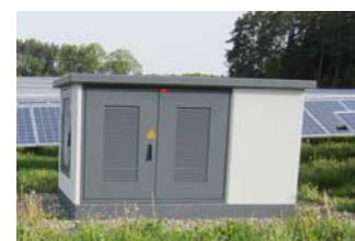
Abb. 12: Trafostation
